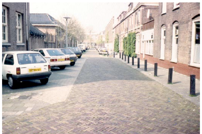
Alternative road materials like cobbles, bricks or coloured tarmac.
