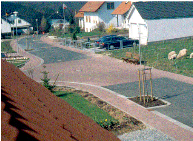
Alternative road materials and 'planters' built out into the road will slow the traffic.
