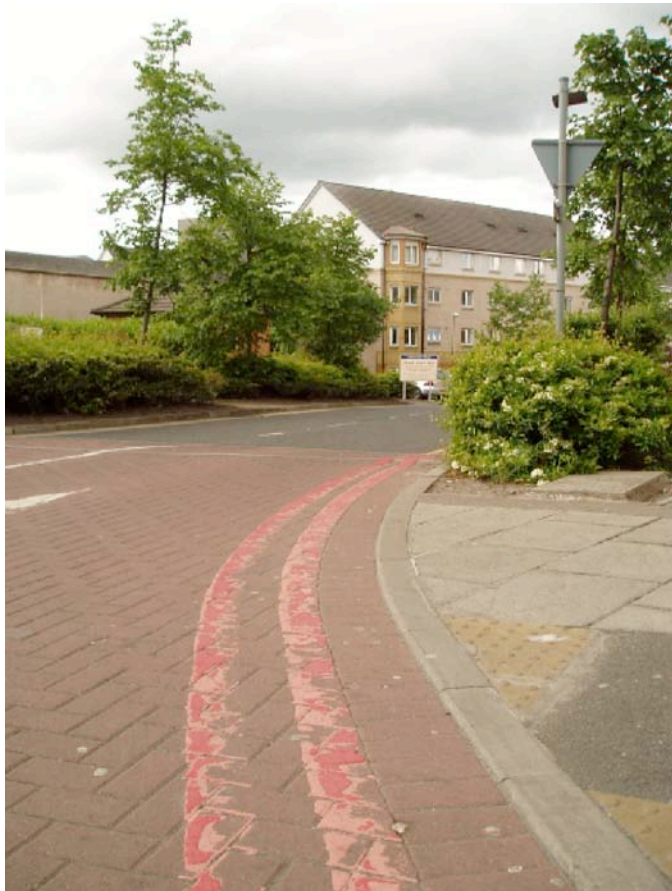
Reduced sight lines using trees or planters.
