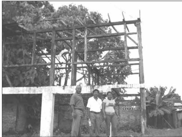
Members of the local action committee in Esmeraldas, Ecuador. A large number of buildings in the town were damaged by a fire caused by an extensive oil spill
