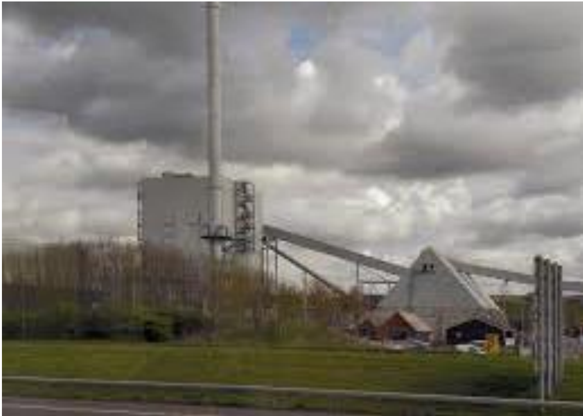
Steven's Croft power station, Photo: David Dixon
