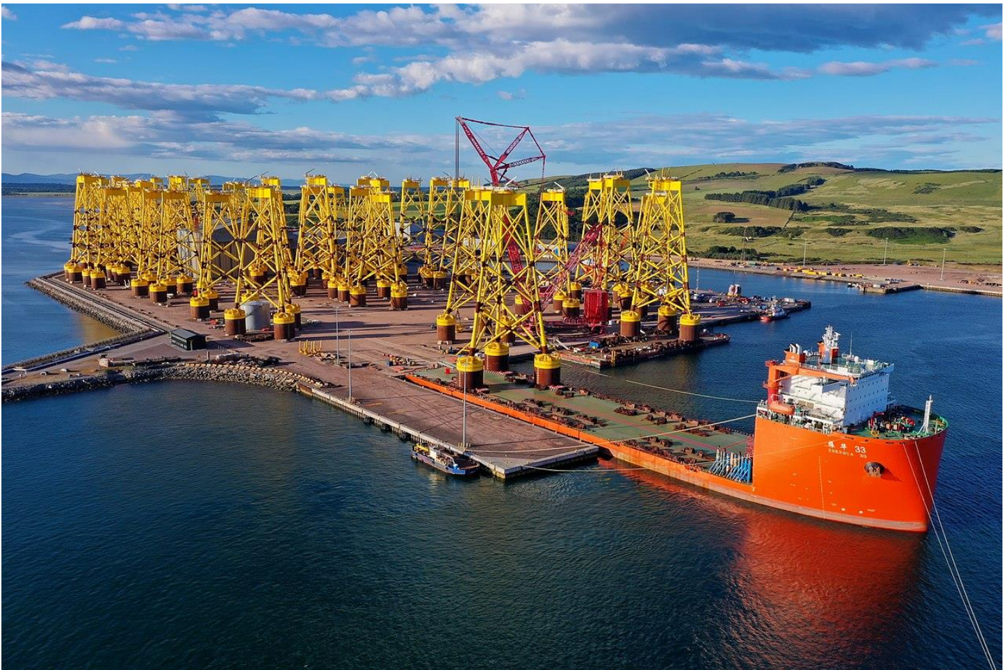
Steel foundations for offshore wind turbines, North East coast of Scotland, 2022. Photo: Zhen Hua, Wikipedia.
